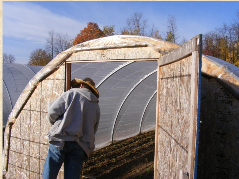
End-wall exterior 1x3's used to frame door and jamb, secure cut ends of plastic cover to end-wall (previously built tunnel)
