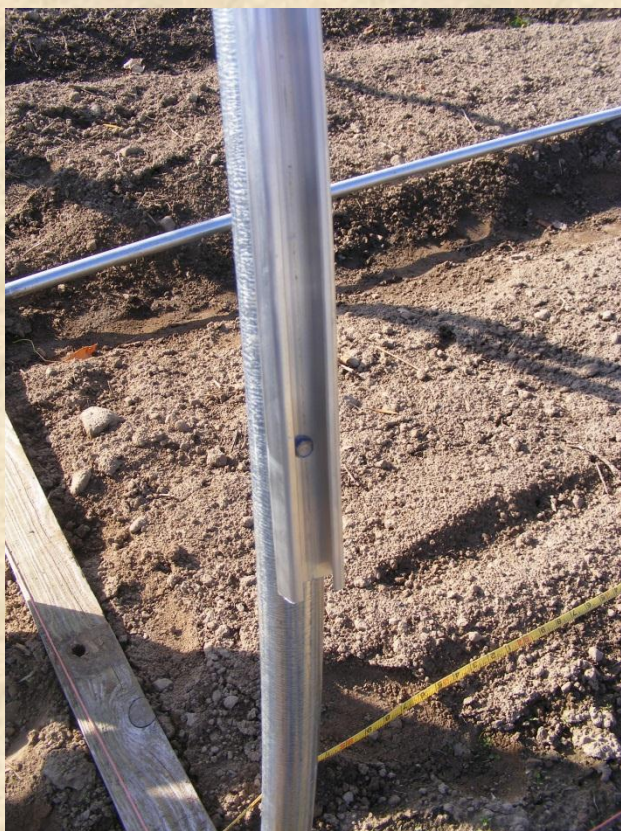
Secured C channel
