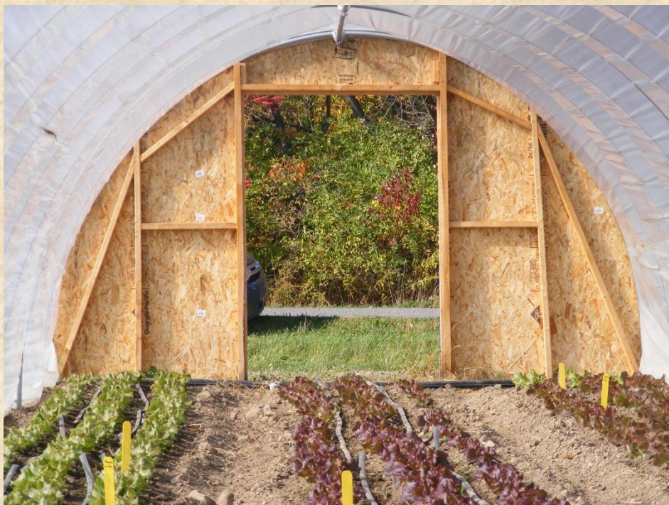
2x3 framed plywood end-wall interior (previously built tunnel)
