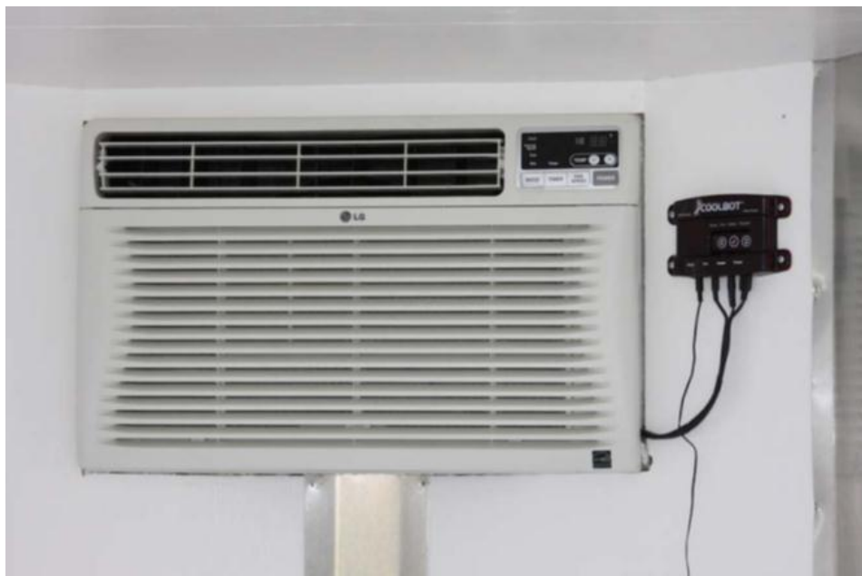
Air conditioner with CoolBot adapter. Photo: NC State Plants for Human Health Institute
