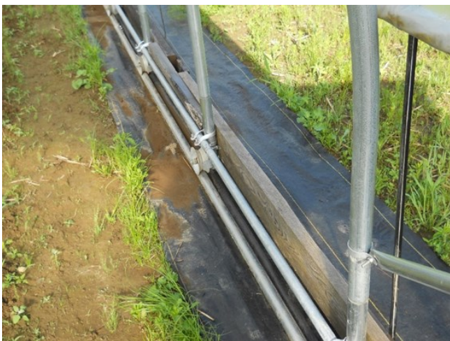
Photo C: When constructing new tunnels, lay ground cloth under the side boards to keep weeds at bay inside and outside the tunnel. Photo ADI
