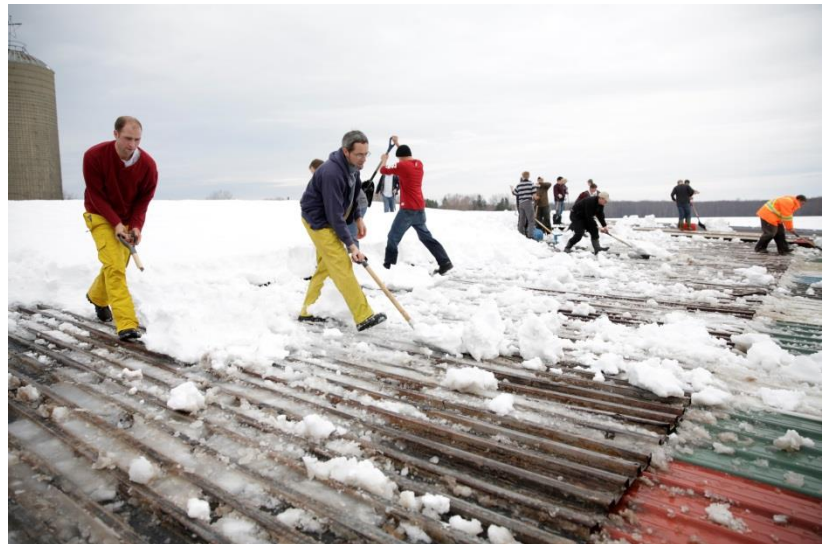
Clearing heavy snow from a barn roof. Photo: Paul Hunt, Mennonite Disaster Service
