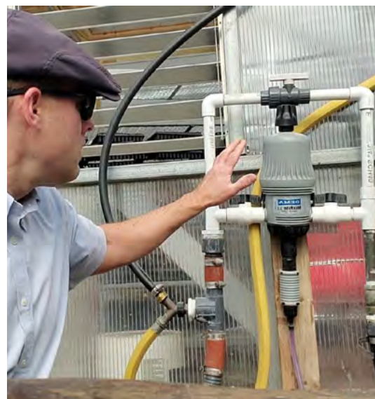
A proportional injector is critical to reduce high pH and alkalinity common in New York irrigation wells. Photo: CCE Cornell Vegetable Program
