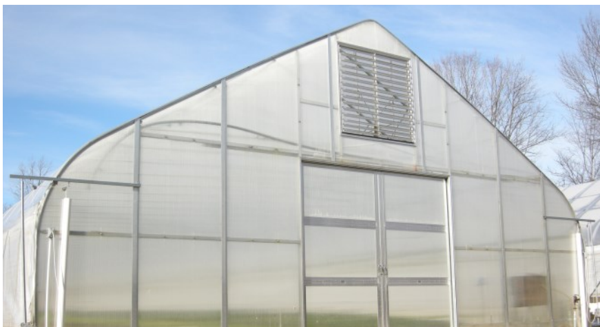
Winter high tunnels need ventilation as shown by the large louver in the gable end.
