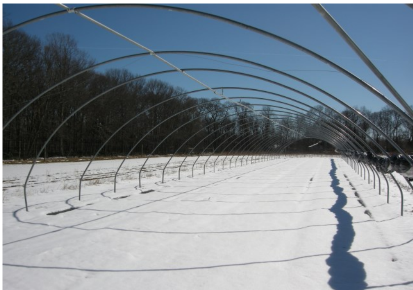
Figure 2. Some high tunnels are designed to have the plastic removed each fall. Photo: Judson Reid, Cornell Vegetable Program
