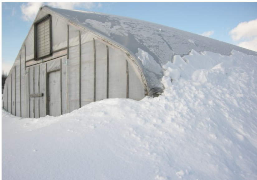
Figure 1. Gothic style structures shed snow best. Photo: Judson Reid, Cornell Vegetable Program
