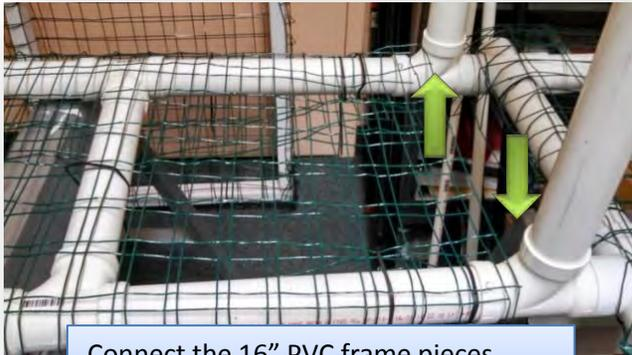
Connect the 16" PVC frame pieces together using the tees, two on a side
