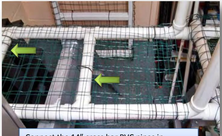
Connect the 14" cross bar PVC pipes in between the side frame to the middle tees.
